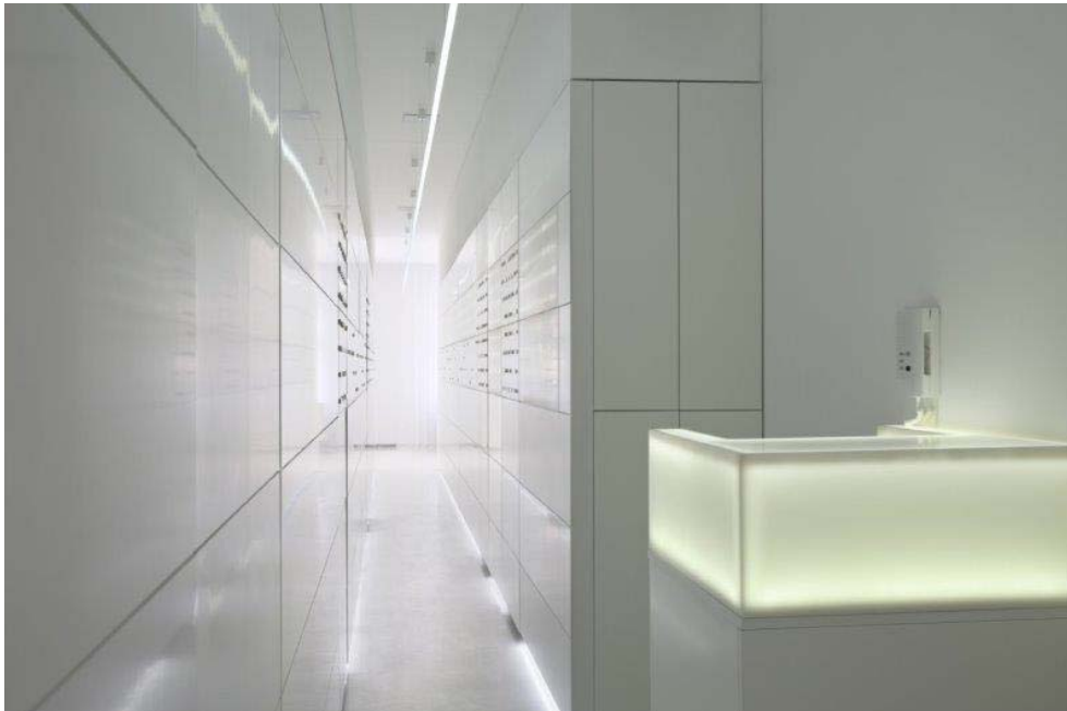
The Dr Dragić Center for Contemporary Laser Vein Therapy in Novi Sad, Serbia. DuPont™ Corian® high-tech surface in the translucent Glacier Ice colour has been used for the backlit wall cladding panels and reception counter; the Glacier White colour of Corian® was used for the door cladding. Project by Studio Fluid; photo Ana Kostić, courtesy of Studio Fluid, all rights reserved.
