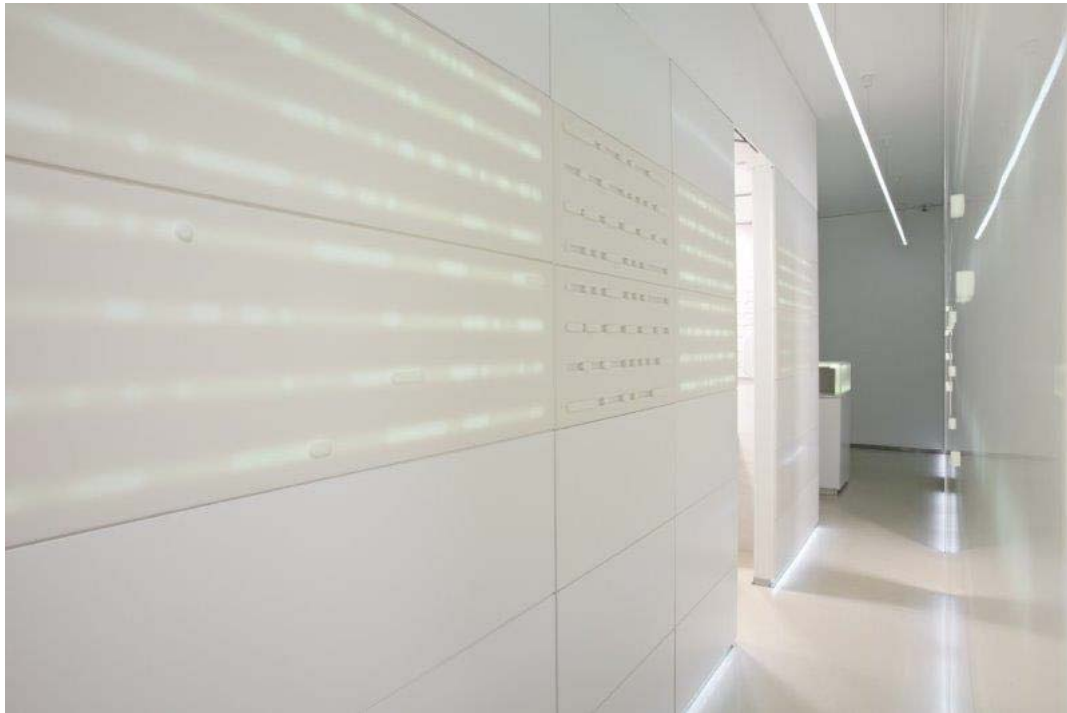
The Dr Dragić Center for Contemporary Laser Vein Therapy in Novi Sad, Serbia. DuPont™ Corian® high-tech surface in the translucent Glacier Ice colour has been used for the backlit wall cladding panels and the reception counter; the Glacier White colour of Corian® was used for the door cladding. Project by Studio Fluid; photo Ana Kostić, courtesy of Studio Fluid, all rights reserved.
